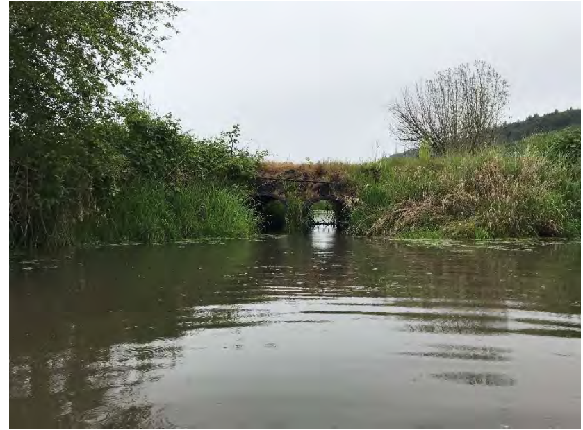
Double arch culvert at Lowe Road crossing
