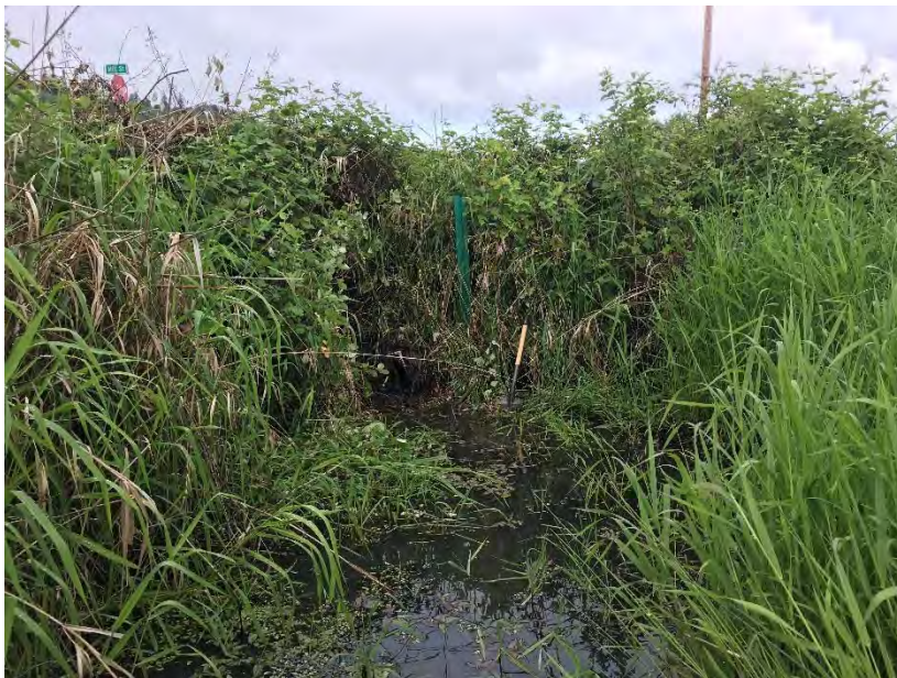
Mill Street culvert, upstream face from channel
