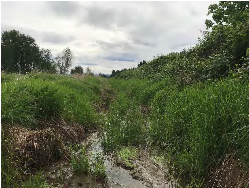
Rock Crest Street culvert, facing upstream from culvert inlet
