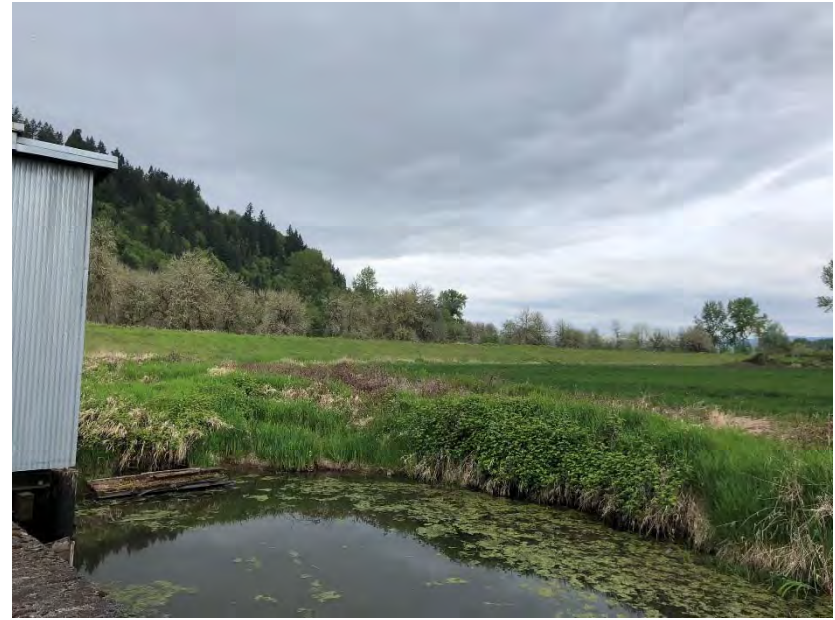
Pump station forebay
