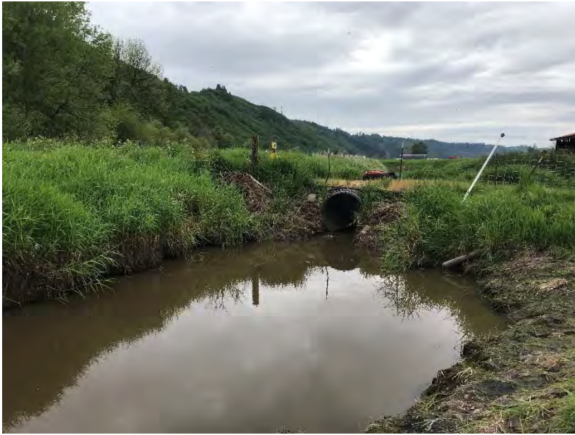
Culvert at Young Road, from upstream right bank
