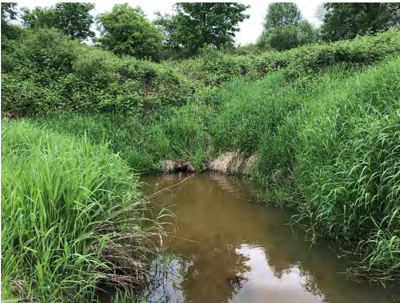
Lewis & Clark Bridge approach road, culvert inlet from left bank
