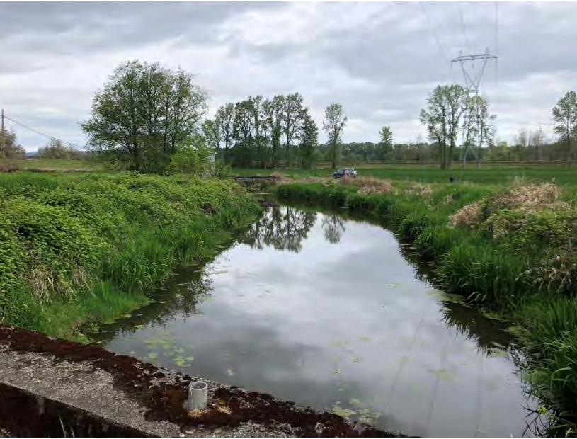
Facing downstream from levee access bridge
