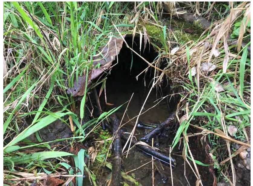
Mill Street culvert, inlet detail
