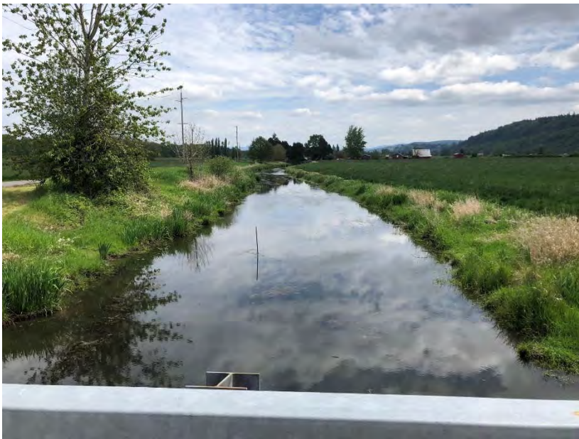
Facing upstream from Amundson Road bridge
