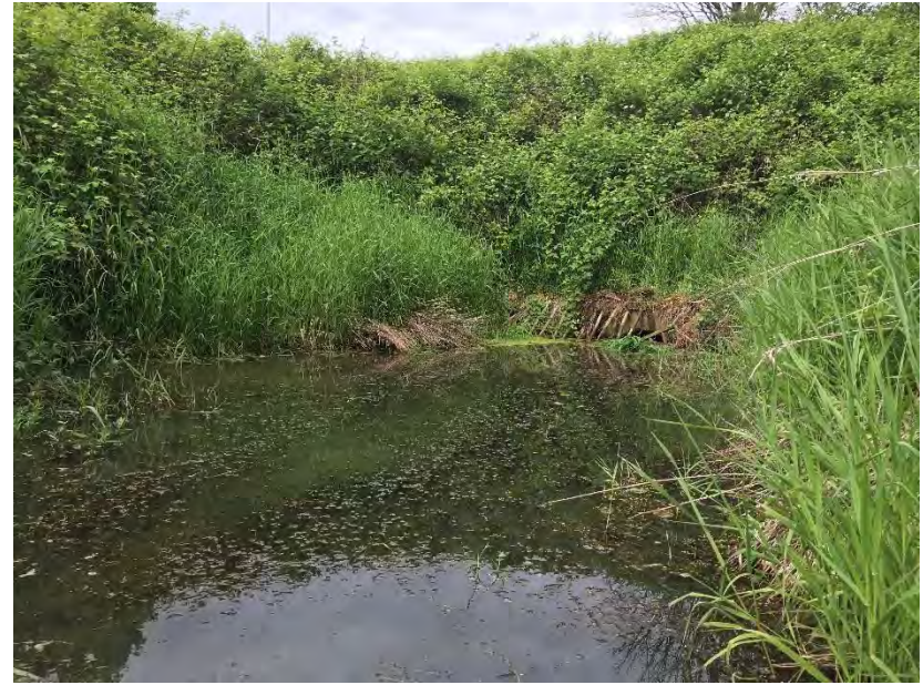
Lewis & Clark Bridge approach road, culvert outlet from left bank
